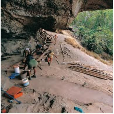
Construction of a boardwalk will protect this Aboriginal art site from inadvertent visitor damage and provide safe access for viewing the art.
